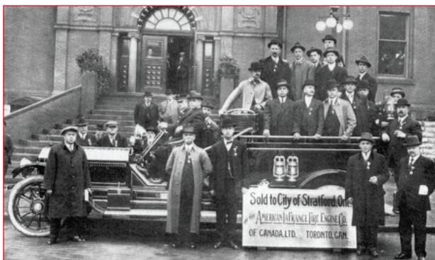
This truck has a gasoline, water-cooled, inline 6-cylinder engine designed by American LaFrance and rated at 104 hp. Power is delivered to the rear drive wheels through drive chains rather than drive shafts as in modern trucks. The original solid rubber tires were later replaced with pneumatic tires, a common practice of the times as tire design improved for better handling.
